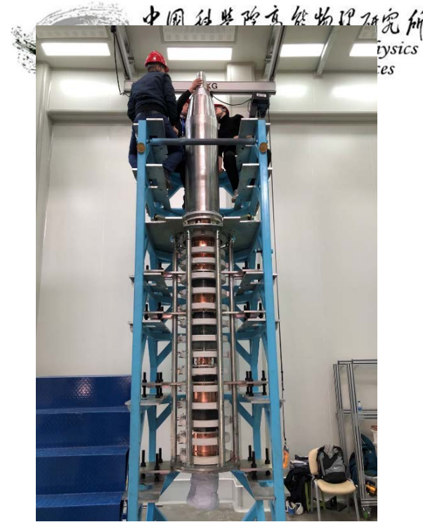
Water jacket installation
