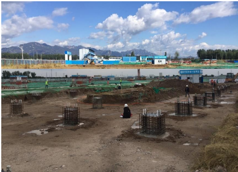
PAPS project being constructed
