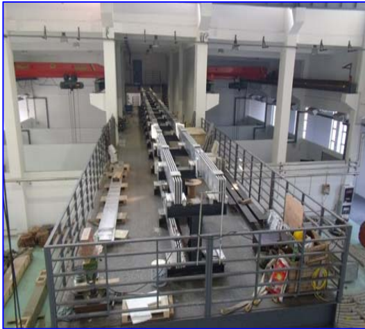
28 MW power supply, deionized water system and the central control system
